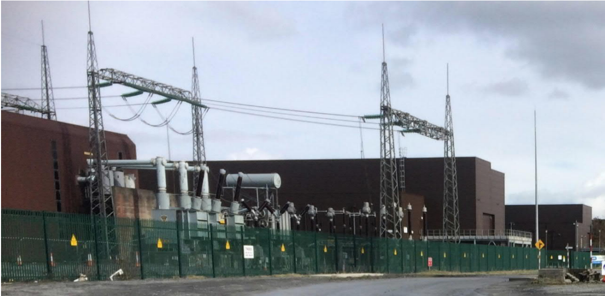
Figure 3.1: Moneypoint 400 kV GIS Substation building
